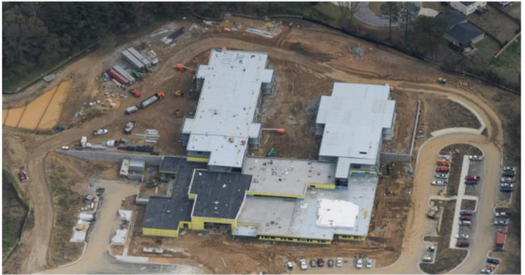
Overall view of building construction progress, from March 2020
