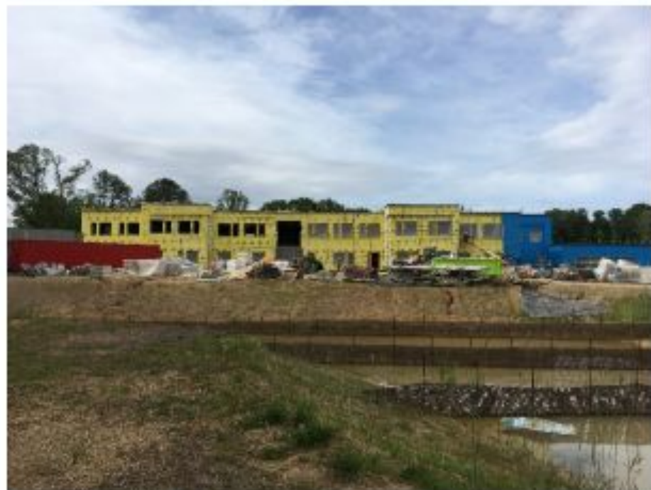
Overall view of Classroom Wing "A"
