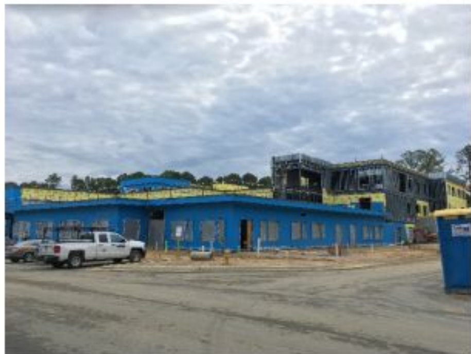
Overall view of Level 1 Admin Wing
